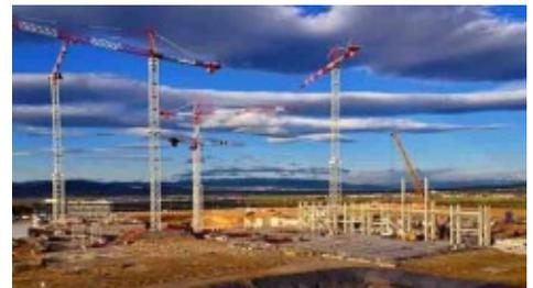
The construction site at Saint-Paul-lez-Durance: when the reactor building is complete, it will rise some 60 metres into the air and reach 10 metres below the ground.
