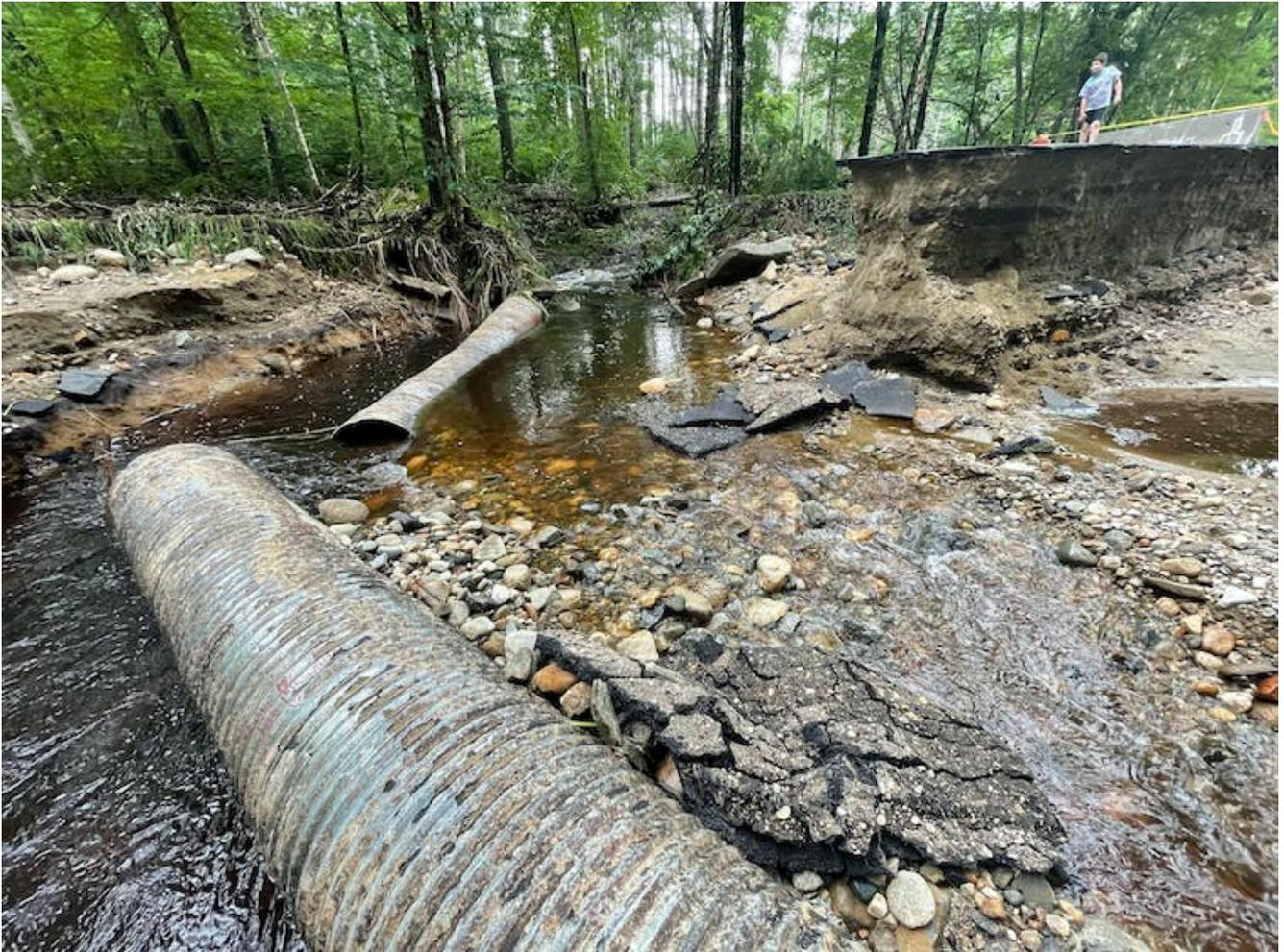
Debris carried by intense rains in July 2021 overtopped a beaver dam (still standing in the background) and washed out this undersized 3-foot culvert in western Massachusetts. It has since been replaced by a more resilient 9-foot structure.
